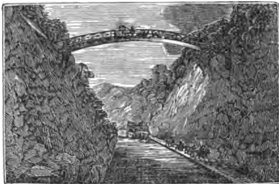
Deep Cut in the Delaware and Chesapeake Canal.
